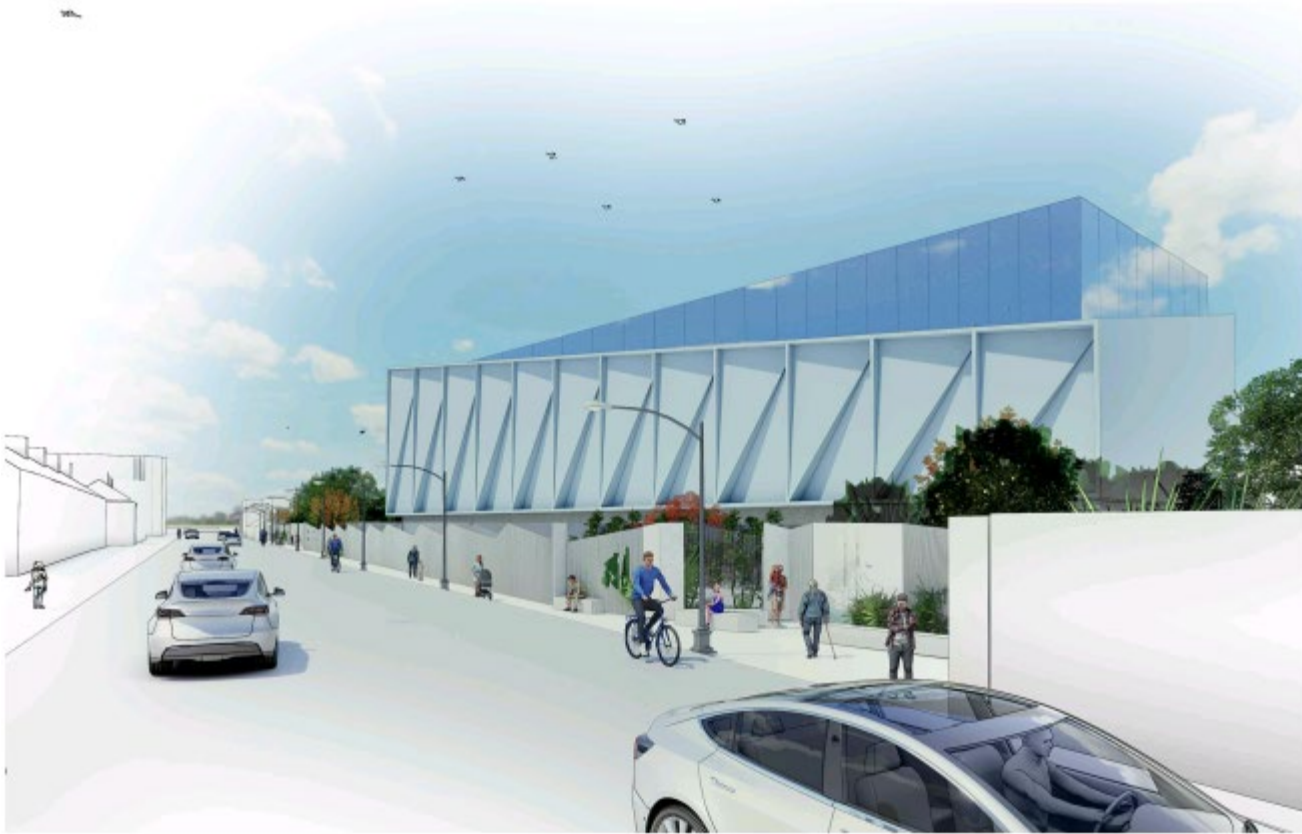
STUDY 1 – Width of precast panels. Panels 5m wide to replicate scale and rhythm of houses on East Wall Road
